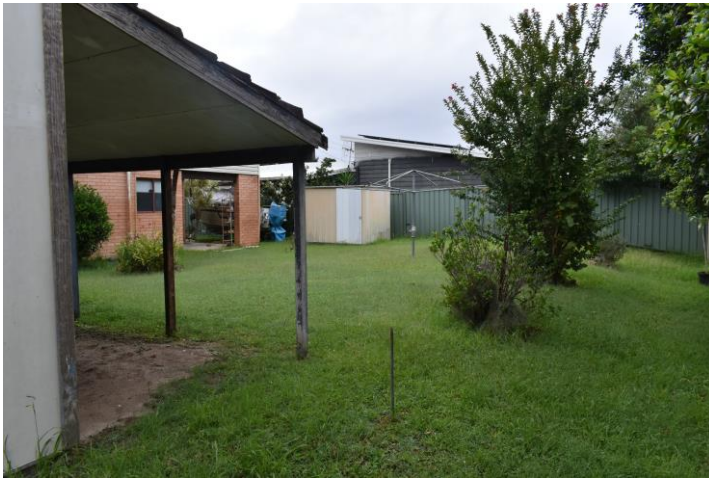
Figure 12: Detail of the soil exposure under veranda area
